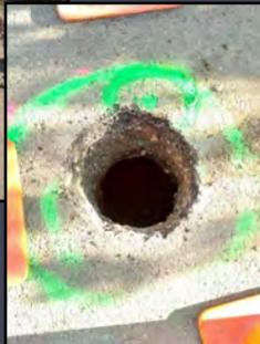
Once it is raised flush with the asphalt a concrete diamond will be poured around the ring and lid to secure it in place.
