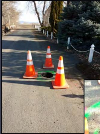
A manhole located on the north side of Hughes Lane was found to be 27" below the asphalt surface of a paved driveway.
