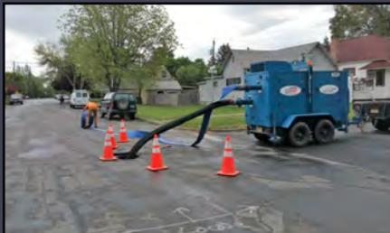
The pump quickly pumped the rain water from the manhole at 1st and "C" Streets east and around the corner to Main Street where the water could run into a catch basin which had already been connected to the new storm line.
