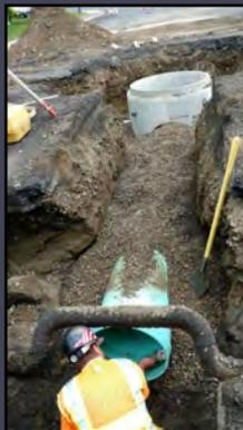
← Another section of natural gas line had to be adjusted so that the new storm line could be installed at the designed grade.
