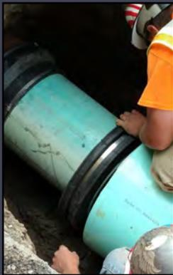
Pictured left, Nate and Brian are connecting the new 21" pipe to the old 15" terra cotta pipe by using special rubber bushings and couplers.
