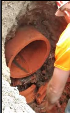
← Brian is using a cutoff blade to remove the bell end of the 15" terra cotta pipe so that a secure connection can be made with the new 21" pipe.
