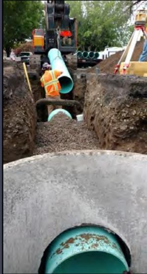
← Here the crew is installing a 21" pipe south from the manhole at the intersection of 1st and "D" Streets.
