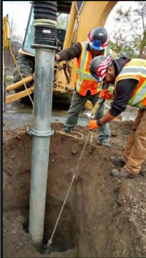
Using the vector truck to carefully hydro-excavate around the brittle terra cotta pipe.
