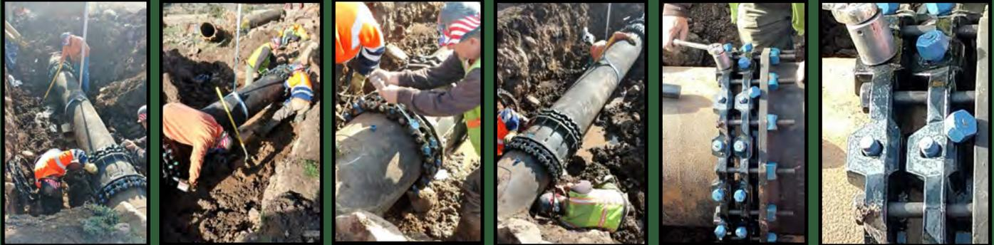
The tandem mega-lugs are designed so that when the specified torque is reached, the huge nut snaps off. There is a smaller bolt bead below the top nut should the mega-lug ever have to be removed.
