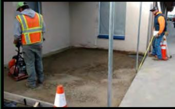
Kris and Nate worked to pour concrete on the north side of the police station. This concrete pad will have an Emergency Electric Generator Unit placed on it.
