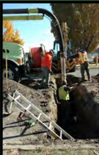
Left: Karl operated the electronic controls while Jake moved the suction tube. Blain operated the high pressure water nozzle to uncover the existing 15" concrete sewer main line.
