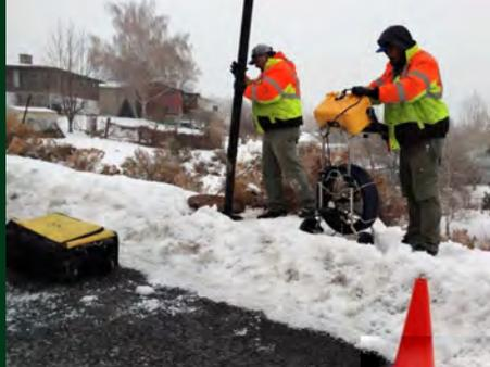
Karl and Jake used the Vivax push-can with the Sonde unit to exactly locate the location of the intersection of two main lines.
