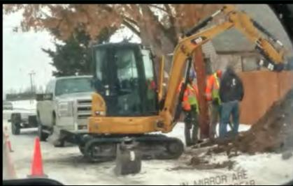
A resident on 5th Street had requested to have their wastewater connection relocated from a substandard line in an undedicated alley, to a main line lying under the 5th Street right of way. Back around 1970, a sewer stub was installed for this purpose. A contractor dug at the described location and was able to find the buried pipe.
