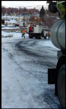
Wastewater was mere inches from overflowing the manhole. Once the vacor truck had successfully removed the wastewater from the manhole, the line was cleaned by forcing the hose to go with the flow.
