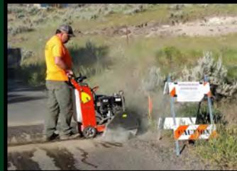
A new wastewater lateral was installed Thursday on Reservoir Road. The chip sealed road surface was saw cut, the 9' deep wastewater main line was exposed, and an insert-a-tee was then used for the new construction.
