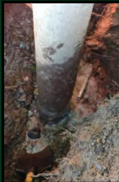
It was a very difficult repair because the water spraying from the pipe was over 80 psi pressure. Water main line valves were partially closed to reduce pressure, but it didn't help much.
