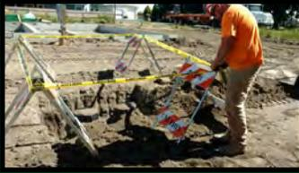
Two new 1" water services were installed this week for the new duplex on 10th Street, which is currently under construction. Here, Nate is using caution tape to prevent vehicles and pedestrians from entering the area.
