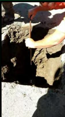
Craig used a water meter key to turn off the corp stop valve.
