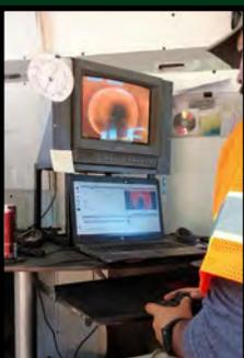
Next, the crew attempted to video-inspect the line. The line was found to be in less than perfect condition with several severe cracks. The pipe was also not perfectly round, causing the camera to become temporarily stuck in the line.
