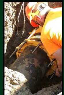
Another water leak near the intersection of Carter and 11th Streets was reported last week. Blain and Brady excavated down to the pipe and sealed the leak. Here, Brady is attaching a bell clamp to the joint.
