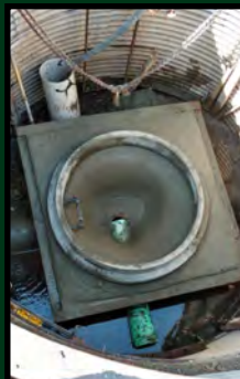
Left: The concrete was placed and formed around the pipes.
