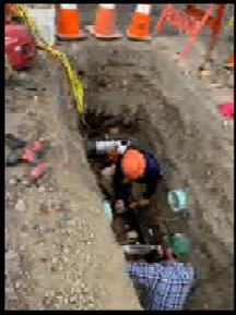
In the Water Department, two separate “hot taps” were performed by a team from the city of LaGrande. A “hot tap” refers to leaving the water main line live while tapping into it for new service.
