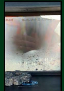
A new residence under construction had a dye test to see if the wastewater line that was installed 15 years ago was still connected into a wastewater manhole near Reservoir Road. The neon green dye shows positive proof that the line is still connected. Next the line was video-inspected. While the inside of the pipe showed some deformities where rocks had made a "dimple" pushing into the pipe, the pipe was found to be in acceptable condition.
