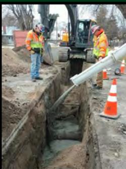
Left: CLSM (low strength concrete) was poured around the other utility pipe crossings to prevent settlement.
