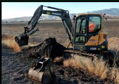
A test pit was excavated last week between the airport and the freeway. The location is very near the crossing of the freeway. Soils were examined by an engineer and ground water depth was measured.
