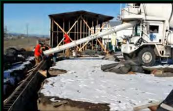
Left: The concrete foundation and stem wall were poured for the pipe shed extension project.
