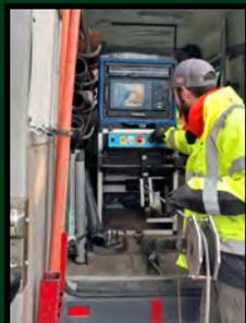
Left: A line between 10th and 11th Streets was video-inspected to determine the cause of a lateral blockage. A pile of roots was found in the main line where a drain cleaner had snaked the line.
