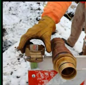
Parts needed to repair the leak near the reservoir arrived this week. The Vactor truck hydro-excavated around the water leak in preparation for the repair work. The brass fitting was installed, the water turned back on and the leak had stopped!
