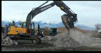
Concrete and asphalt chunks were crushed last week for recycle use on upcoming city projects.
