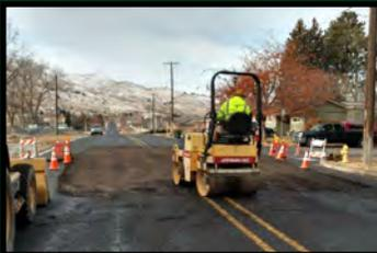
A temporary ramp was then built using asphalt grindings. Vehicles can easily drive over the ramp at a slightly reduced speed. Things will be placed back to normal once the water is no longer needed.
